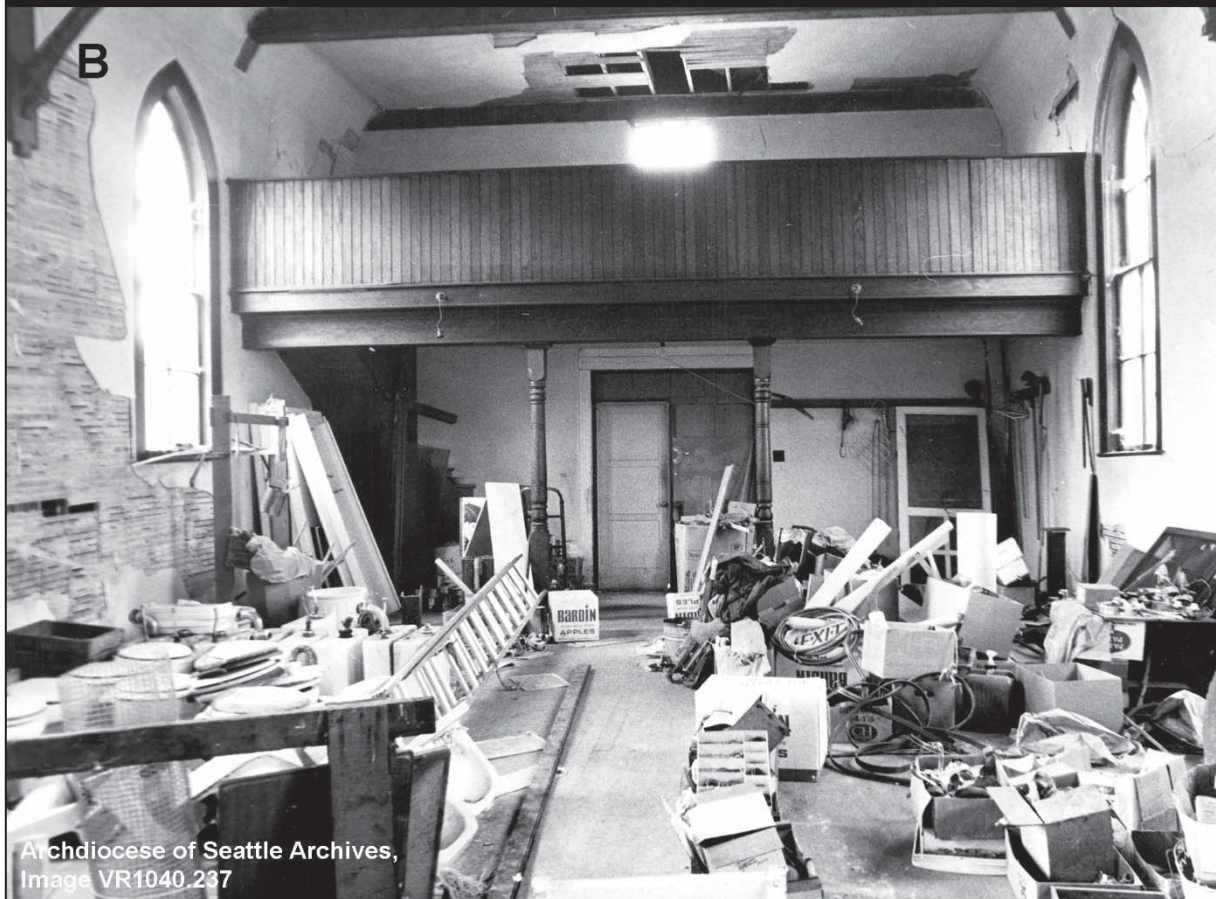
Figure 22. Demolition of the buildings began in 1971 and the remaining furniture and other reminders of the school's past were removed prior to construction of the Gethsemane Cemetery, ca. 1972.
