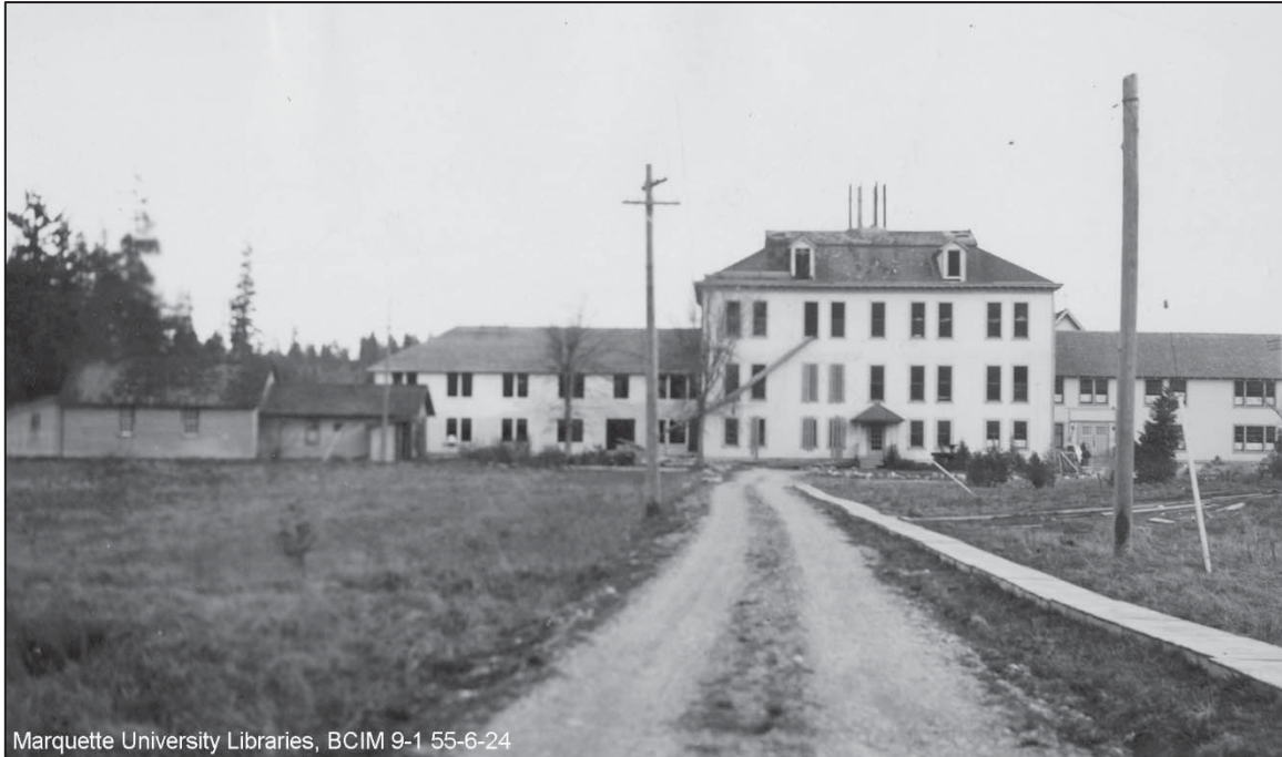
Figure 16. Construction of new buildings nears completion, ca. 1933.
