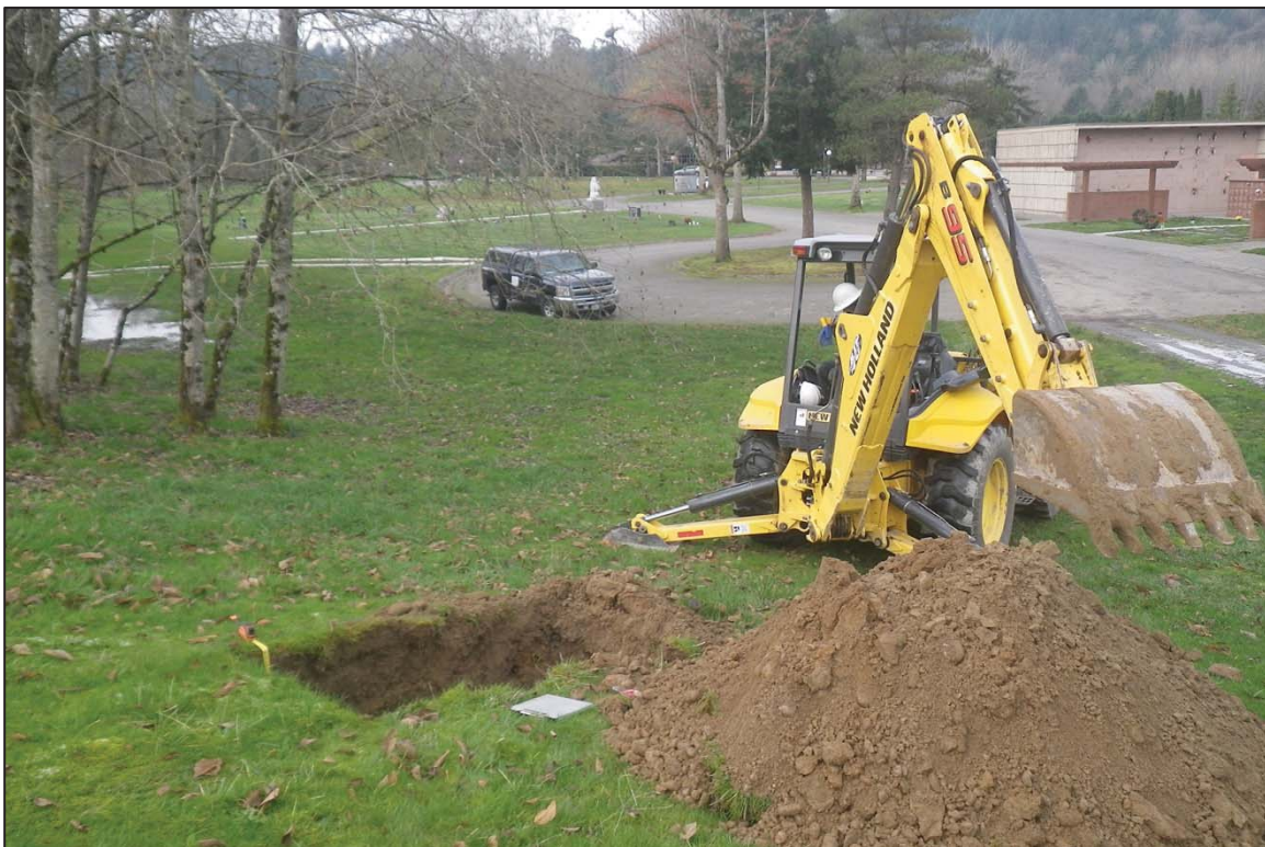
Figure 4. Overview of test pit excavation, showing Test Pit (TP) 3 at the toe of the artificial berm, view southwest.
